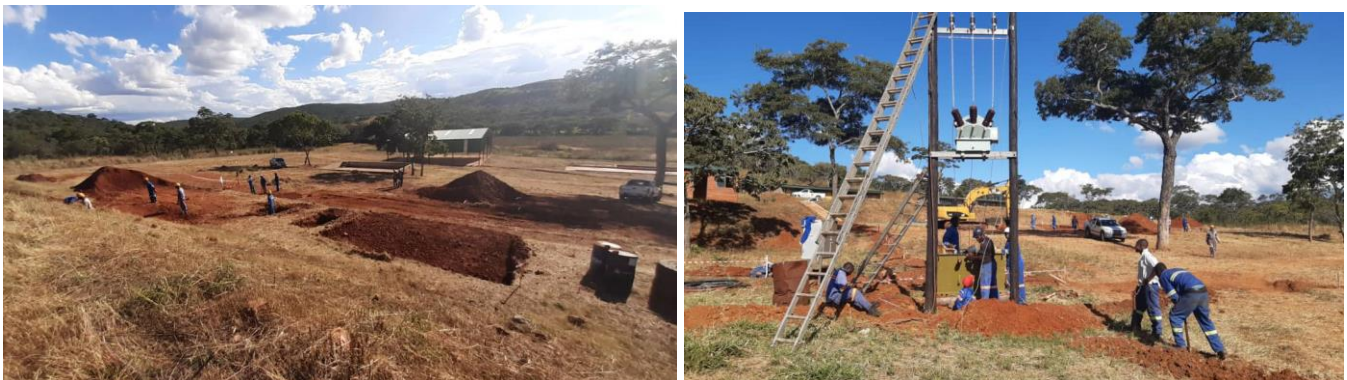
Figure 1 & 2 – Civil works for crushing plant and installation of power transformer
