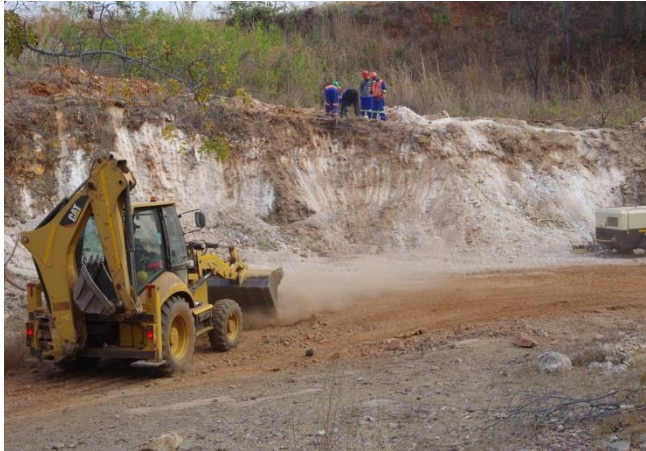
Preparing for the first blast
