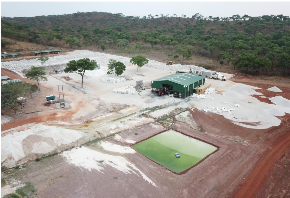
Figure 1 –Arcadia Pilot Plant
